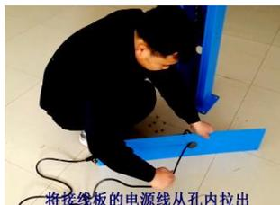
11. Exit the power supply terminal block plug
